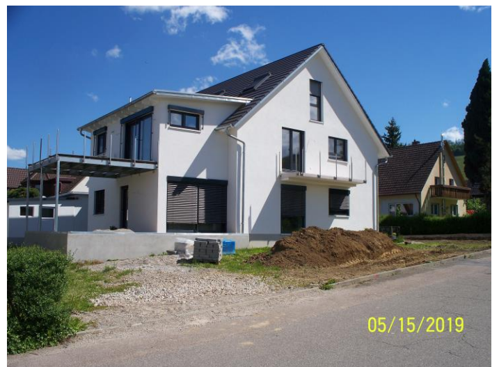
Home Being Remodeled
